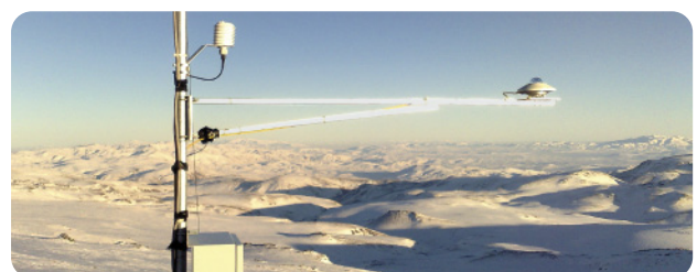
Installation on Erzurum Palandöken Mountain
